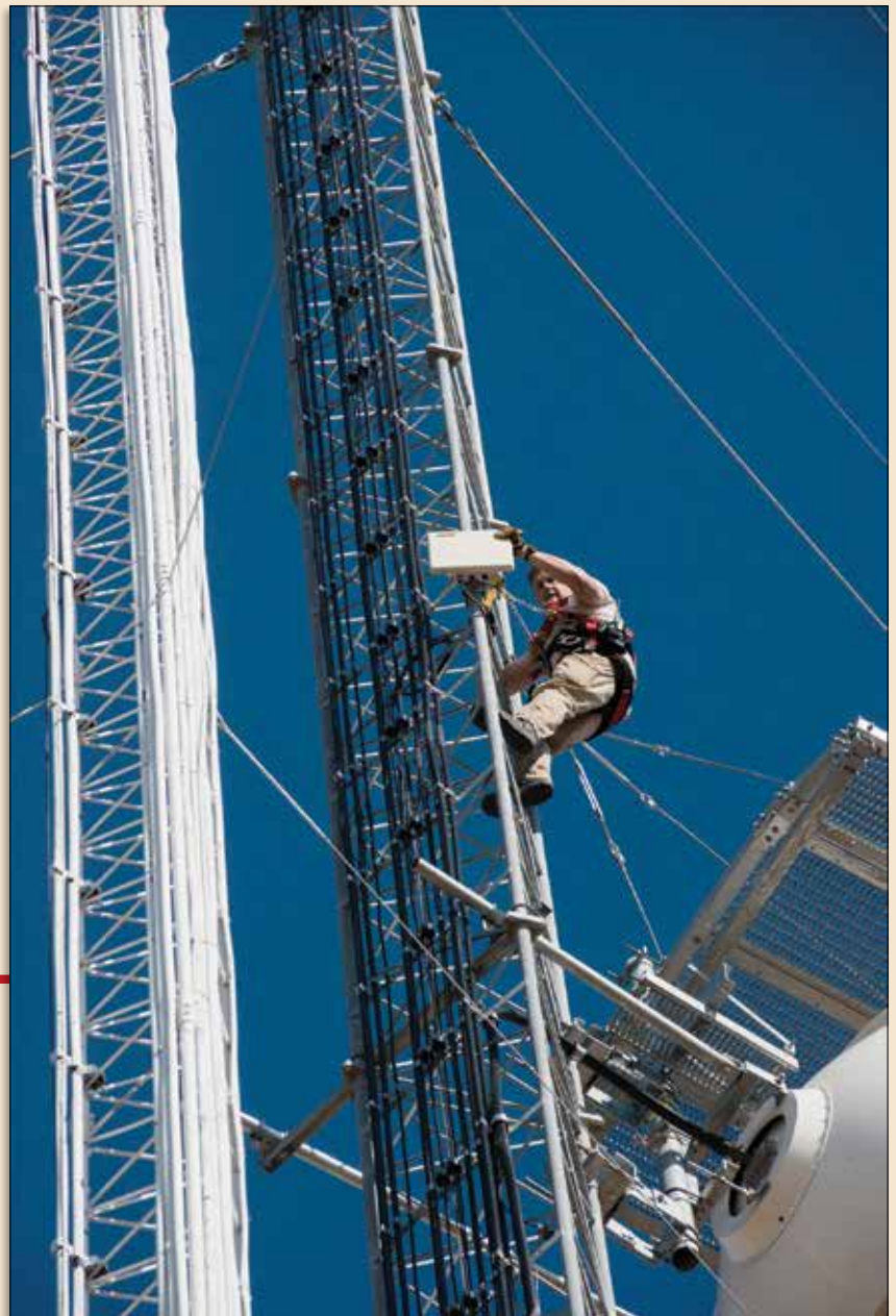
Shane Brown, Emergency Communications & Preparedness Program Manager, conducting cell tower maintenance.
