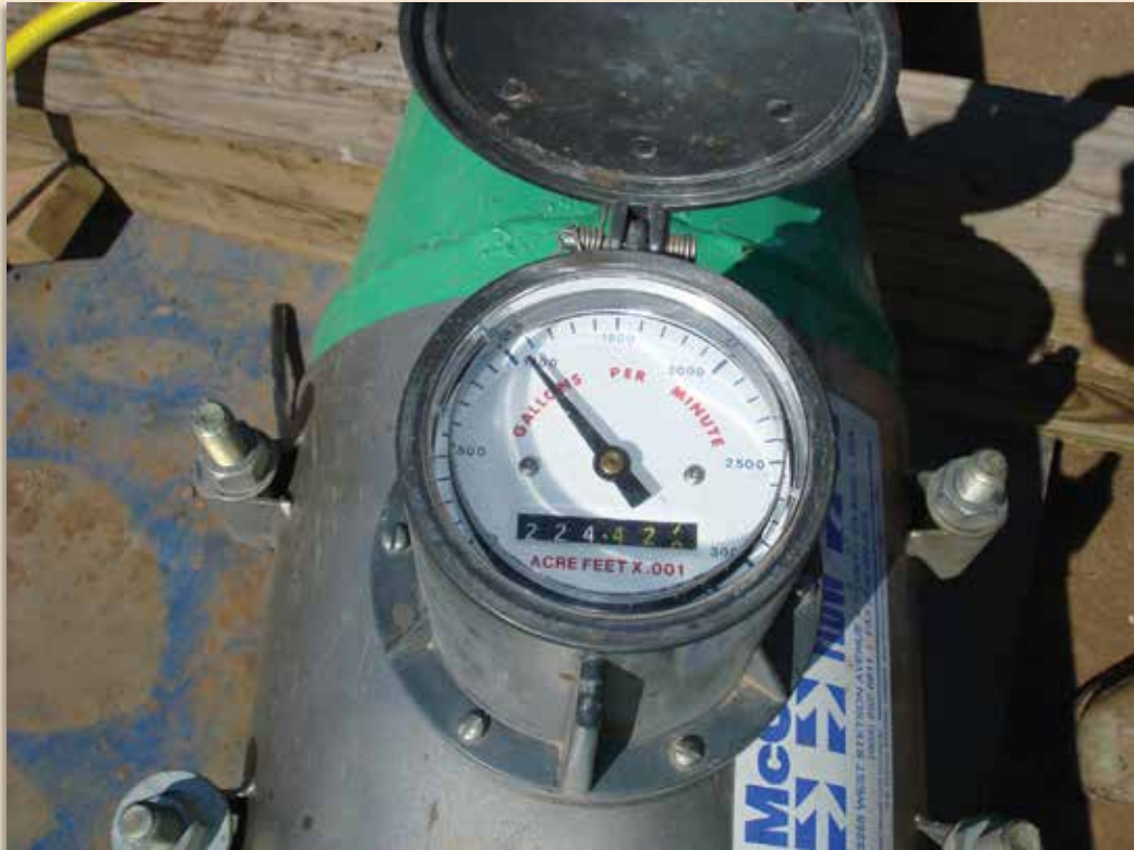
Metering and measuring water use helps to analyze saving opportunities and prevent water waste. Metering has been a strategy in each of the water plans.
