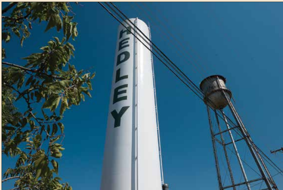
In 1987 the City of Hedley was awarded CDBG funding to build a new standpipe. Thirty-two years later, in 2019, the City received funding to have that standpipe refurbished and painted.
